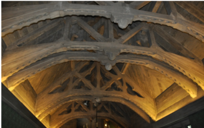
Figure 5 - Concrete Trusses in the Sylvester House
